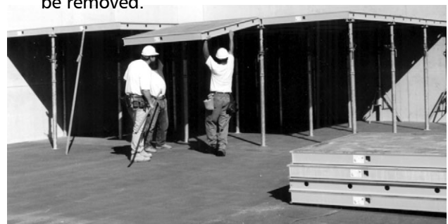
Typical crew is three workers.
