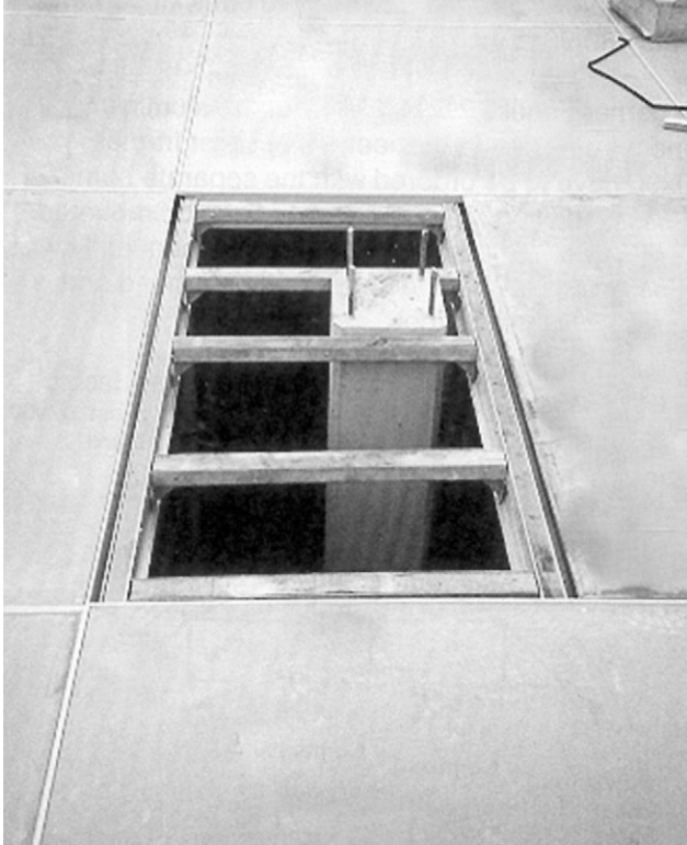
Adjustment Beams and Transverse Beams ready for plywood installation
